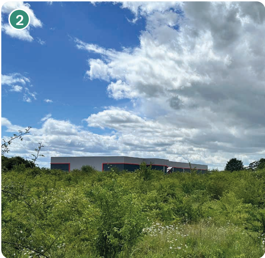
View facing towards Salvation Army Unit
