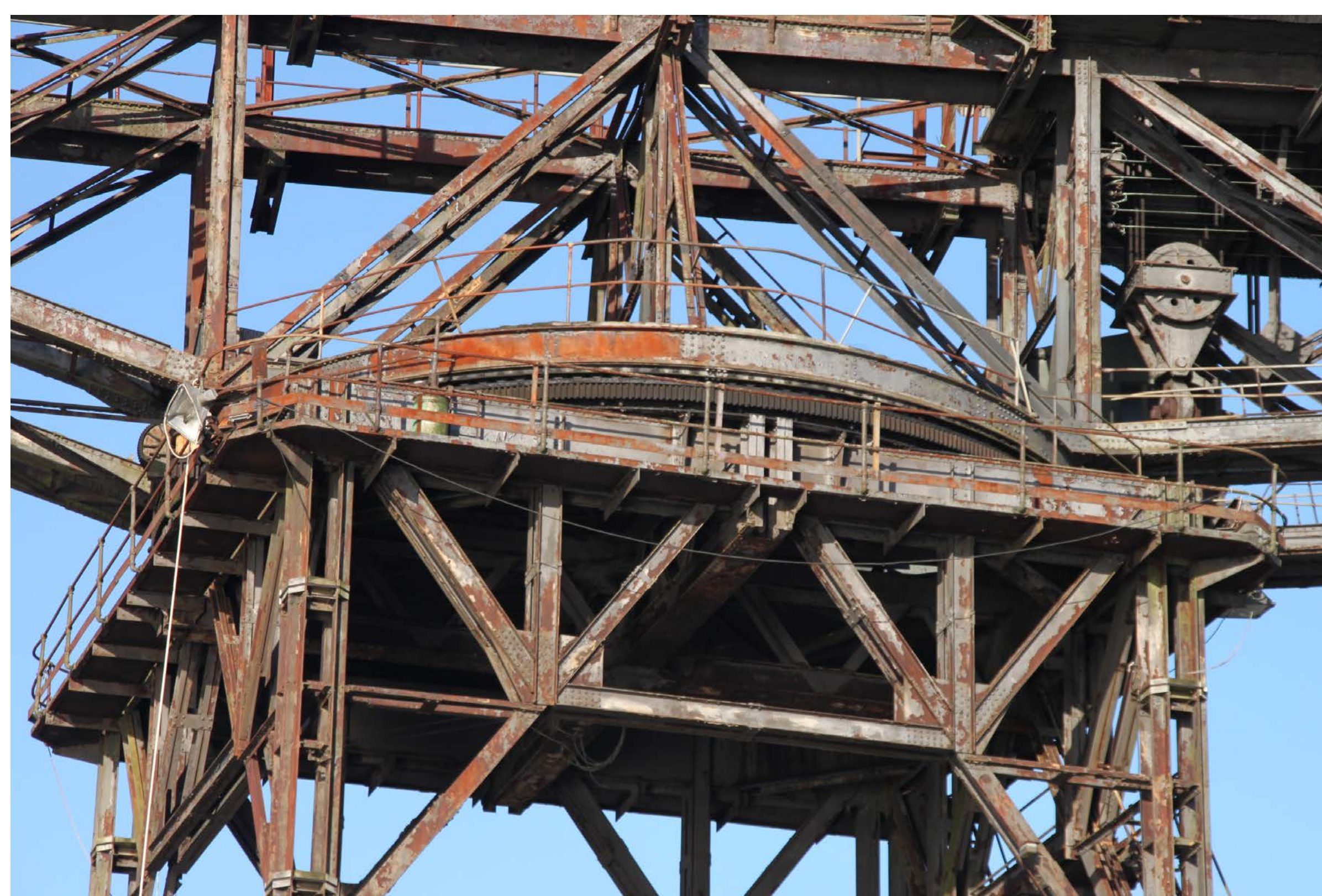
Crane structure in need of refurbishment
