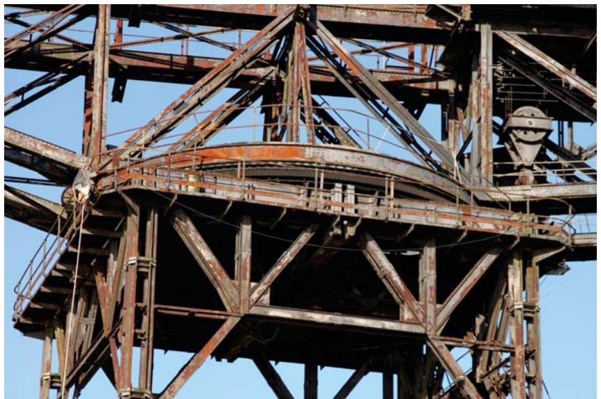
Crane structure in need of refurbishment
