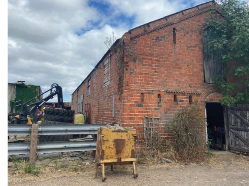
5. Existing barn to be retained and restored
