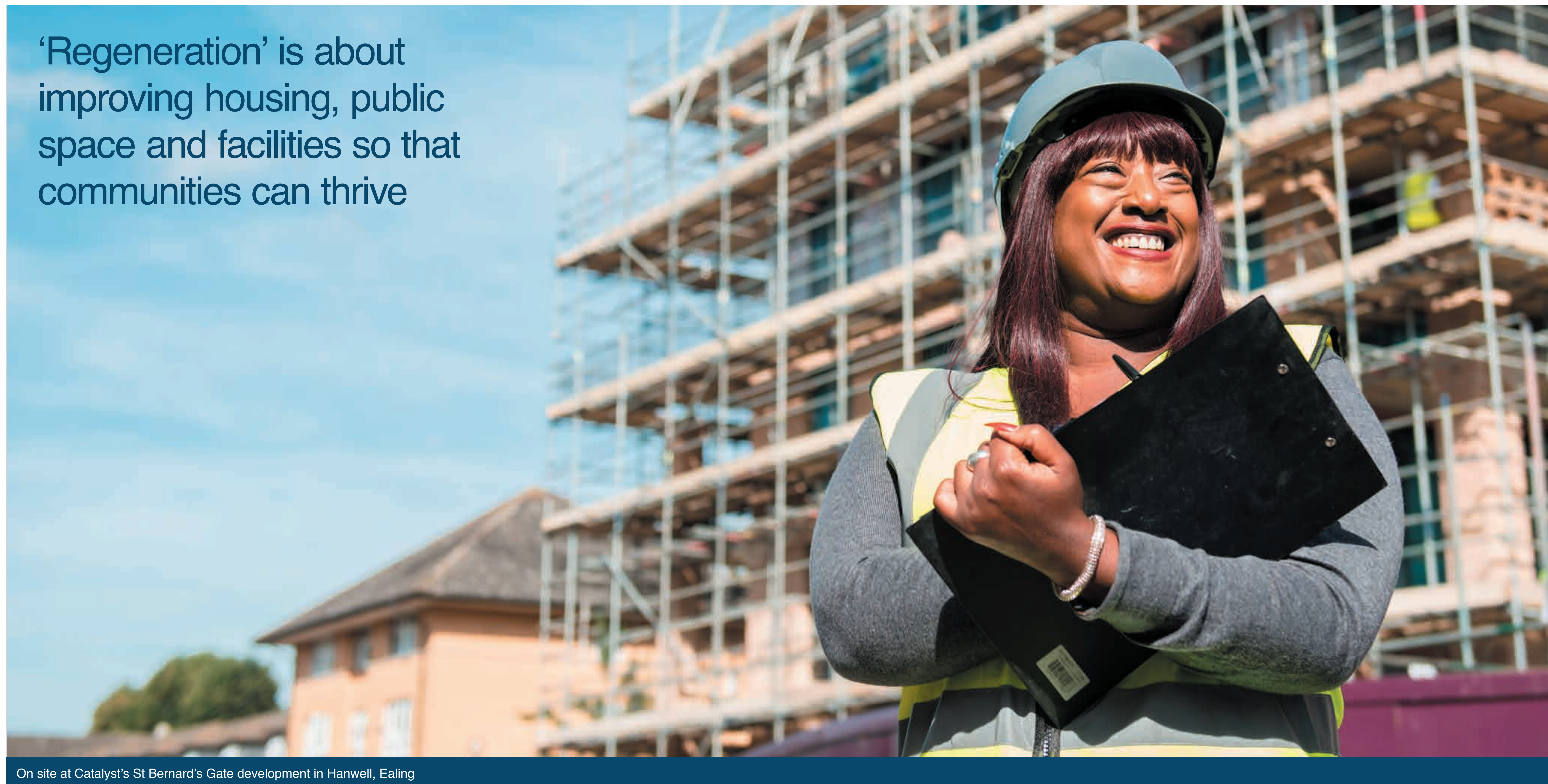
On site at Catalyst's St Bernard's Gate development in Hanwell, Ealing
