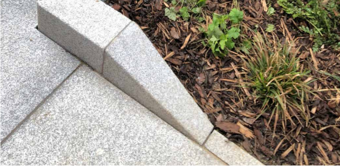
Dropped kerb junctions or kerbs edges with gaps for runoff to filter through
