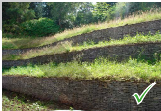
Gabion walls where vertical faces are necessary
