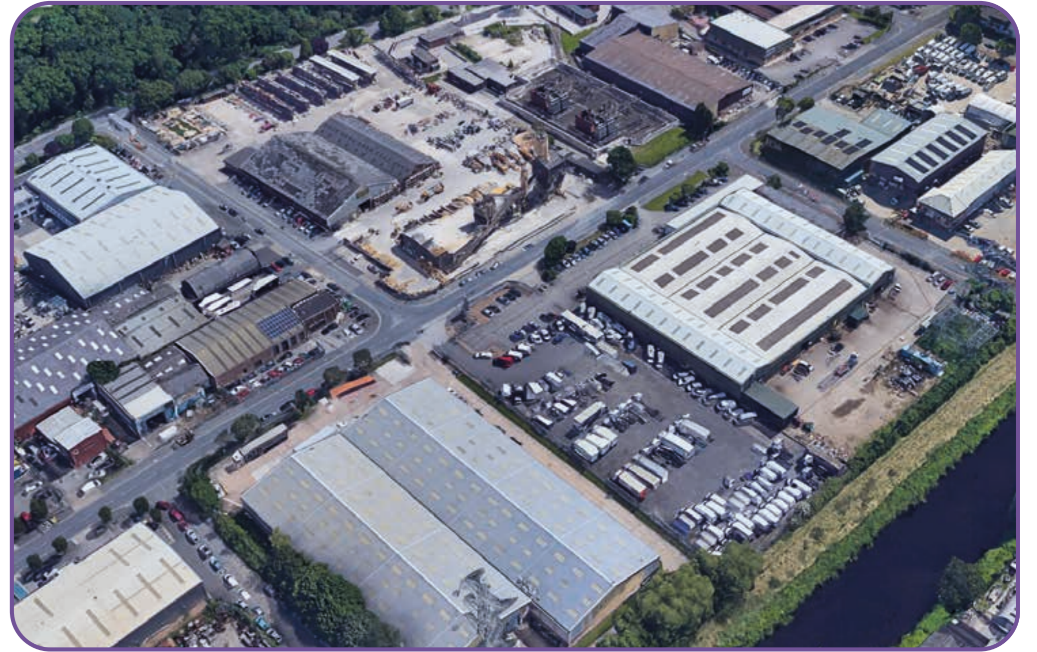
Industrial/Commercial Area, Brighouse - Aerial View
