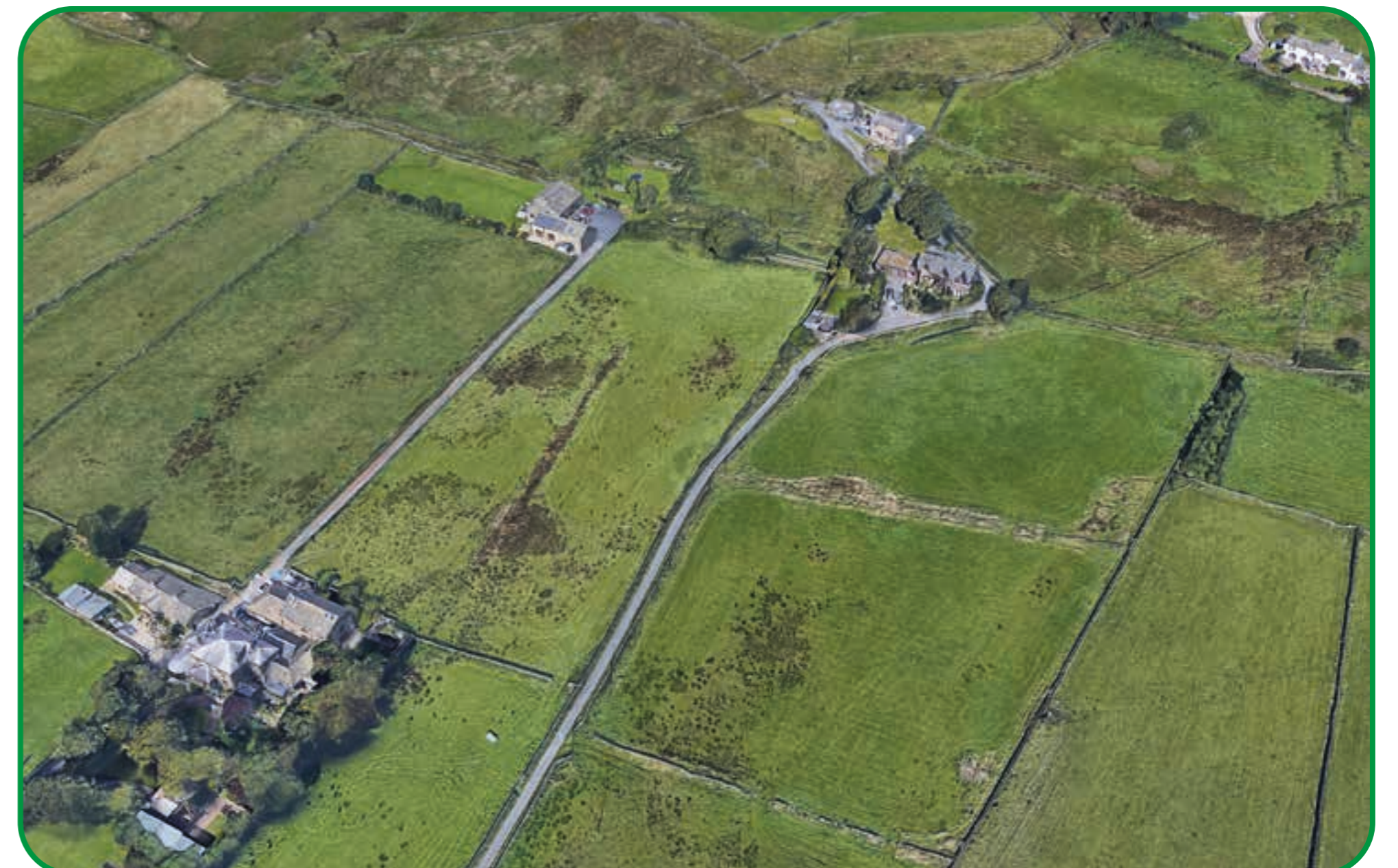
Homes accessed via Bradshaw Lane
