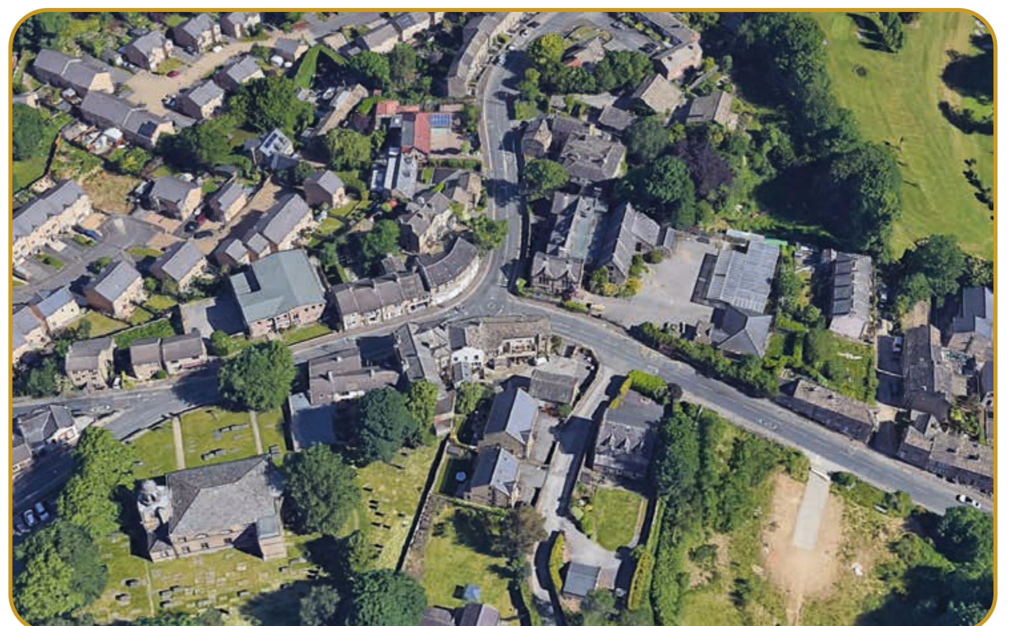
Ogden Lane/ Church Street, Brighouse
