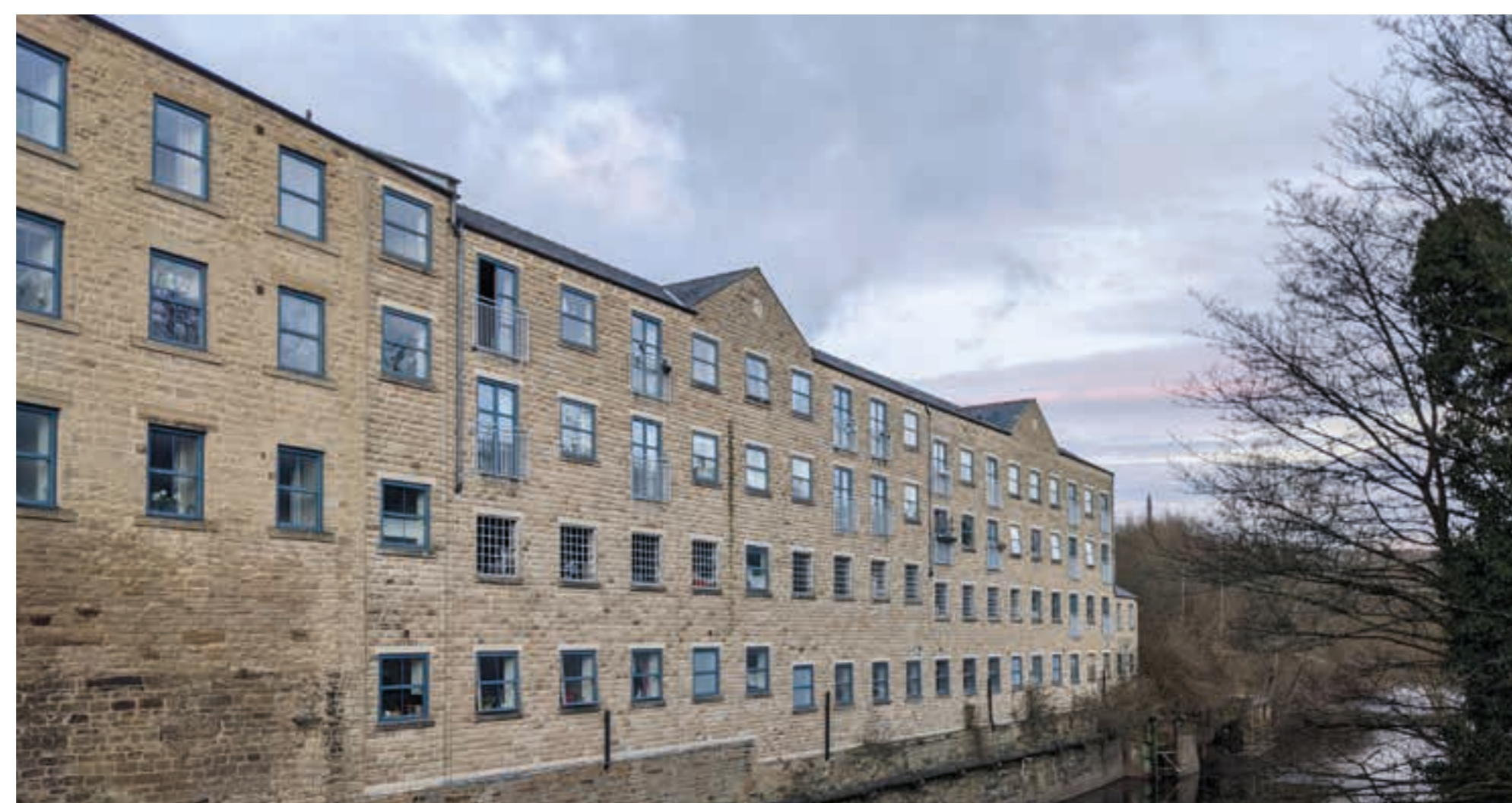
Old Cawsey, Sowerby Bridge
