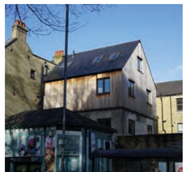
The Vault, Hebden Bridge
