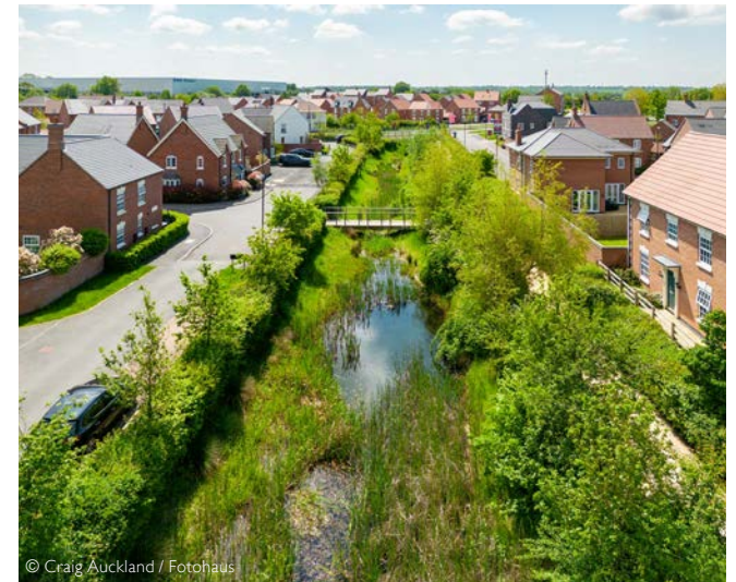
Large swales incorporated into green corridors
