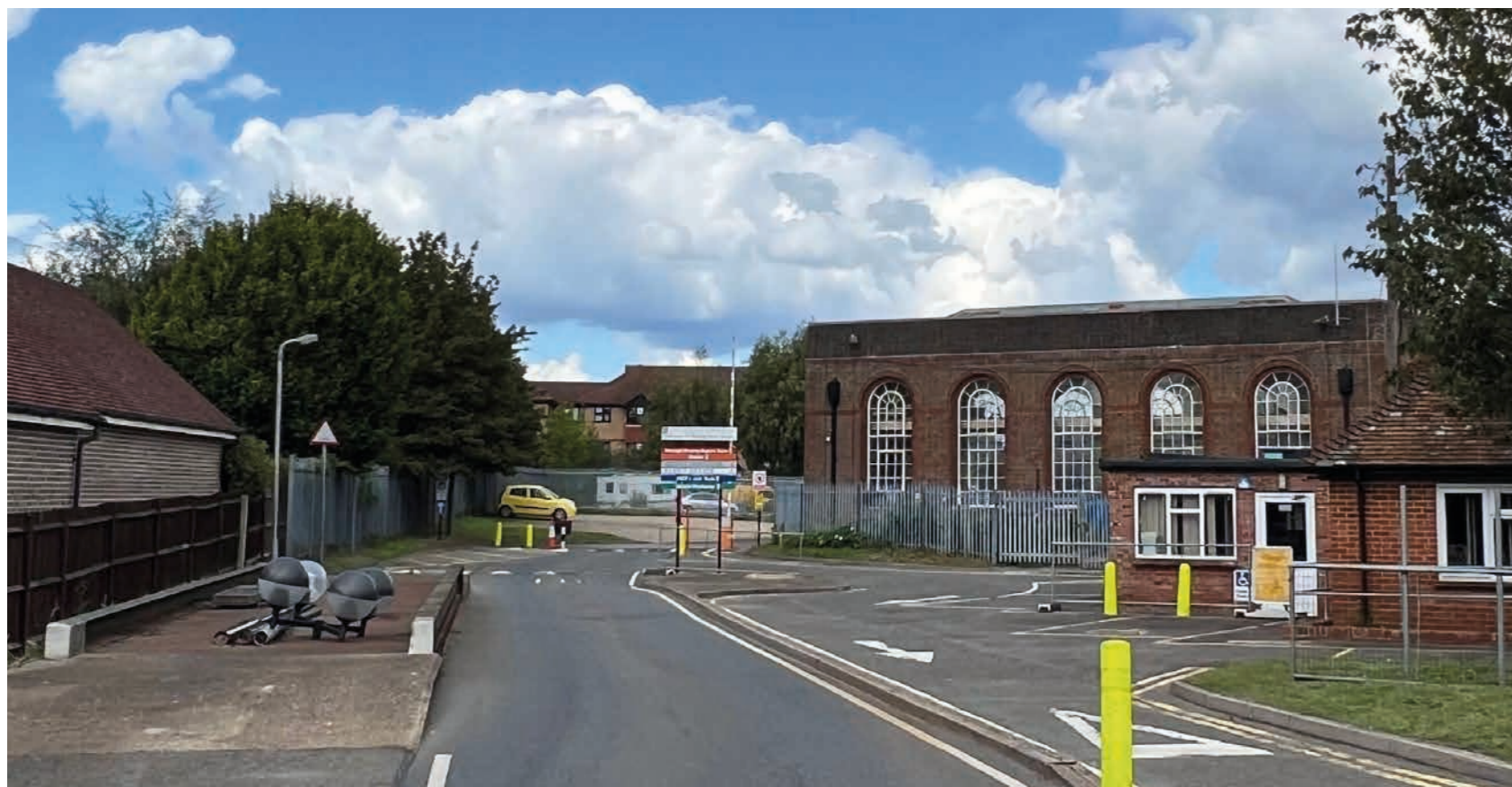
South site entrance looking towards victorian pump house
