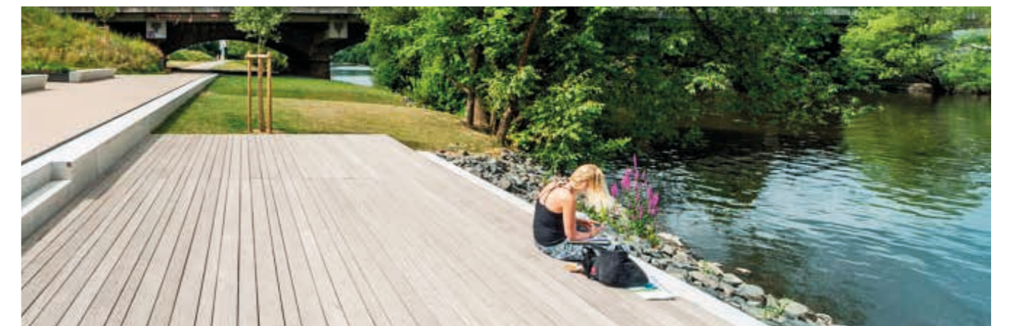
Riverside viewing platform
