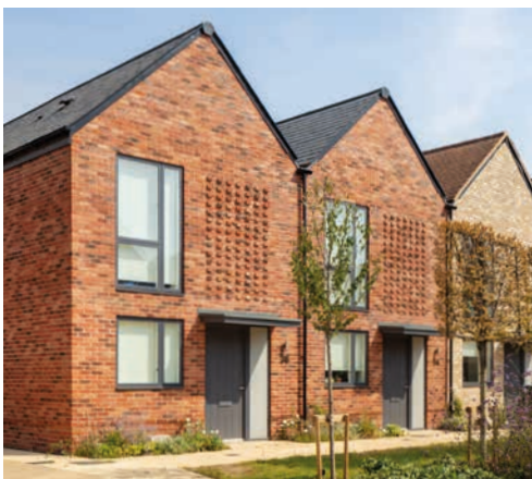
Example of a terraced typology with distinct character created through varied brick colours, interesting roof form and brick detailing
