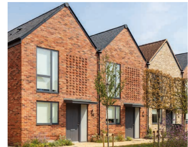
Conventional house types with minimal changes of brick tones but character achieved through brick detailing.
