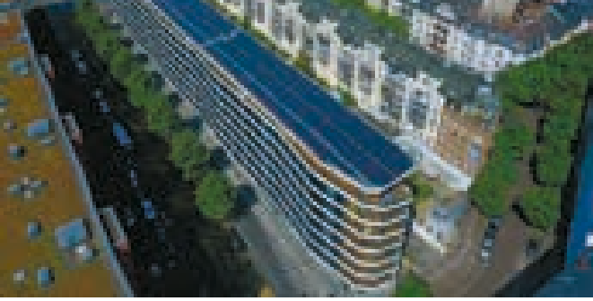
Green buildings - Rooftop PV panels, and PV facades (Active-Cityhouse Frankfurt a. M., Photo Herbert Kratzel)
