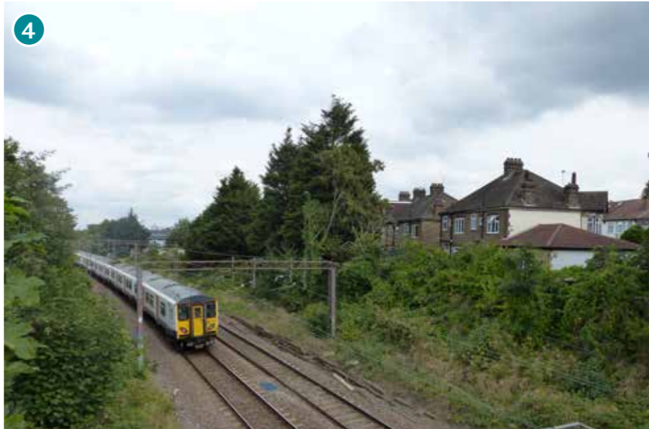
Adjacent railway lines
