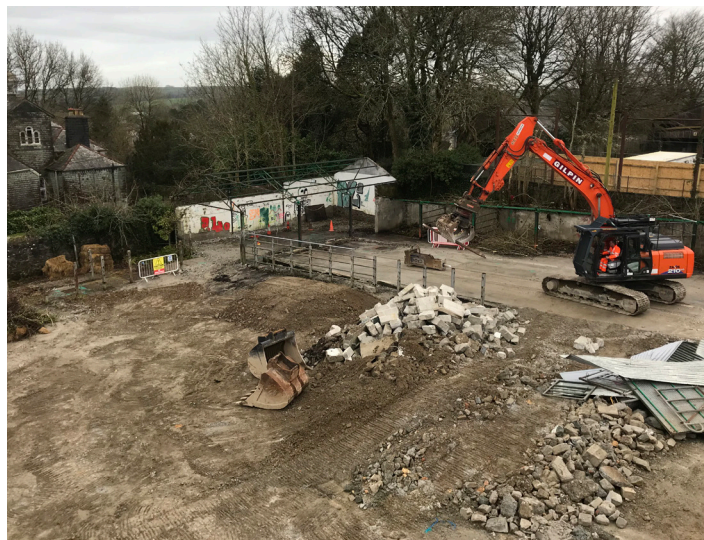
Demolition in January 2021
