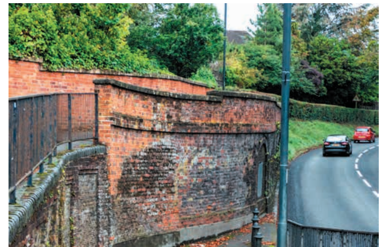
4 Castle Hill bridge
