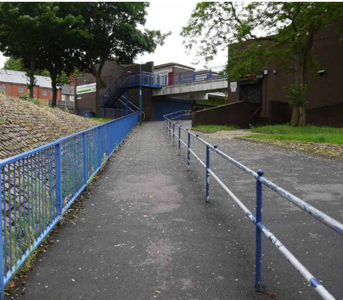
A ramp up from the underpass leads to Church Square, a shopping parade which has seen better days.
