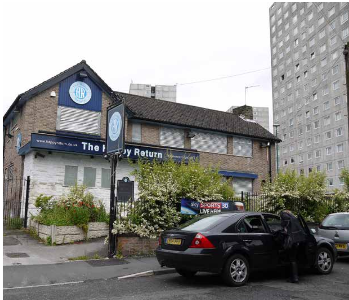
Redevelopment of the Happy Return Pub is an opportunity to create an attractive gateway to the site from the south west
