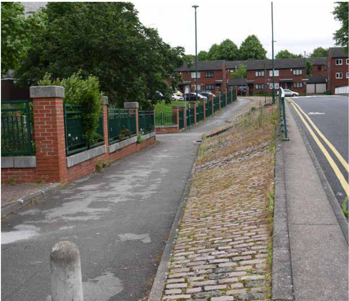
The carriageway of Church Street has been elevated in an arrangement that separates pedestrians and vehicles. Whilst this was intended to protect pedestrians the result is an unnecessary barrier to movement as traffic is reasonably light in this area.
