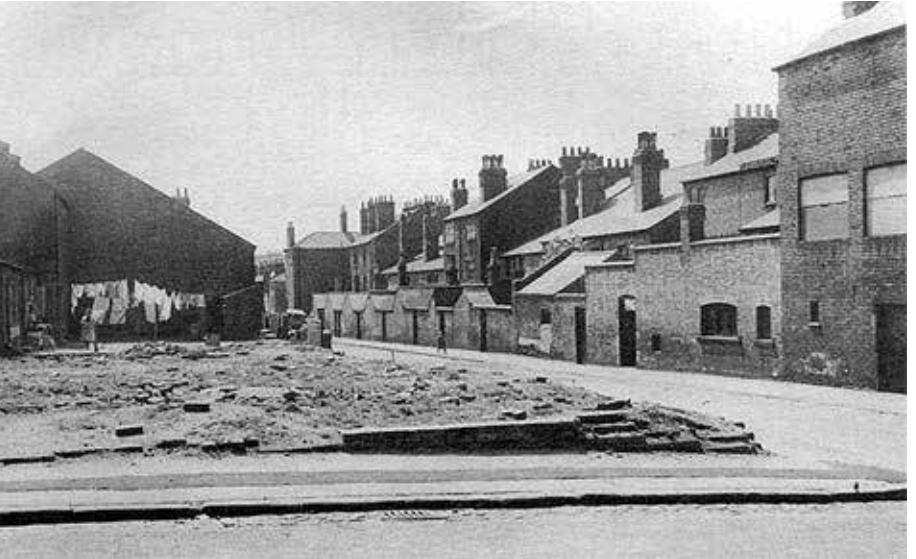
6. Gable end of former Lenton Picture Palace during demolition of Tyne Street in 1961. The building was rented to Edward Peat & Son's Beehive Mills until December 1911 when it was acquired by A P Lowe Ltd, a lace embroidery manufacturer, who stayed there until the building was demolished in the 1960s.
