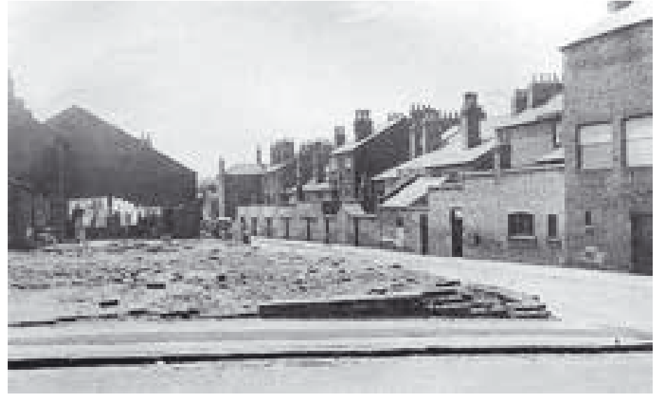
6. Gable end of former Lenton Picture Palace during demolition of Tyne Street in 1961. The building was rented to Edward Peat & Son's Beehive Mills until December 1911 when it was acquired by A P Lowe Ltd, a lace embroidery manufacturer, who stayed there until the building was demolished in the 1960s.
