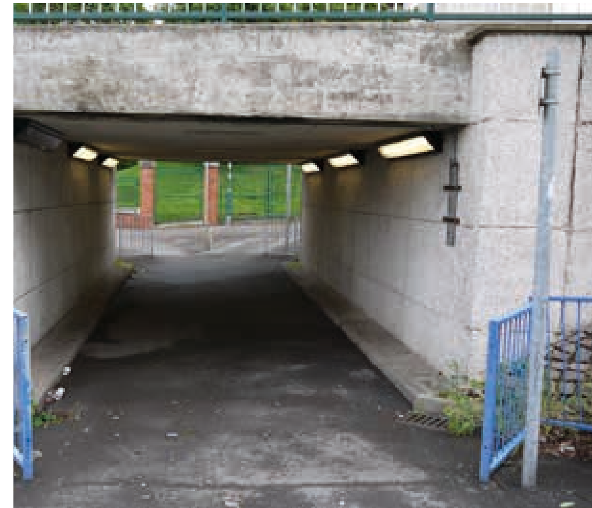
The underpass below Church Street is intimidating, particularly after dark.
