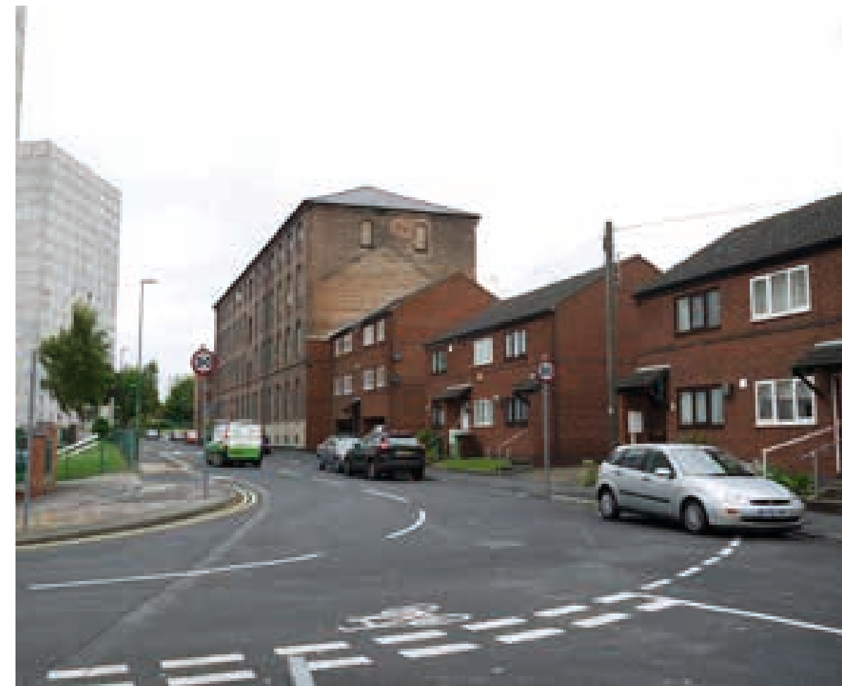
Simpsons, now converted to student residences is a part of the area's industrial heritage and a local landmark.
