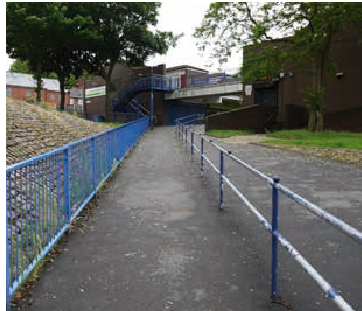
A ramp up from the underpass leads to Church Square, a shopping parade which has seen better days.
