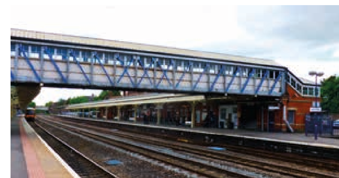
Existing station bridge
