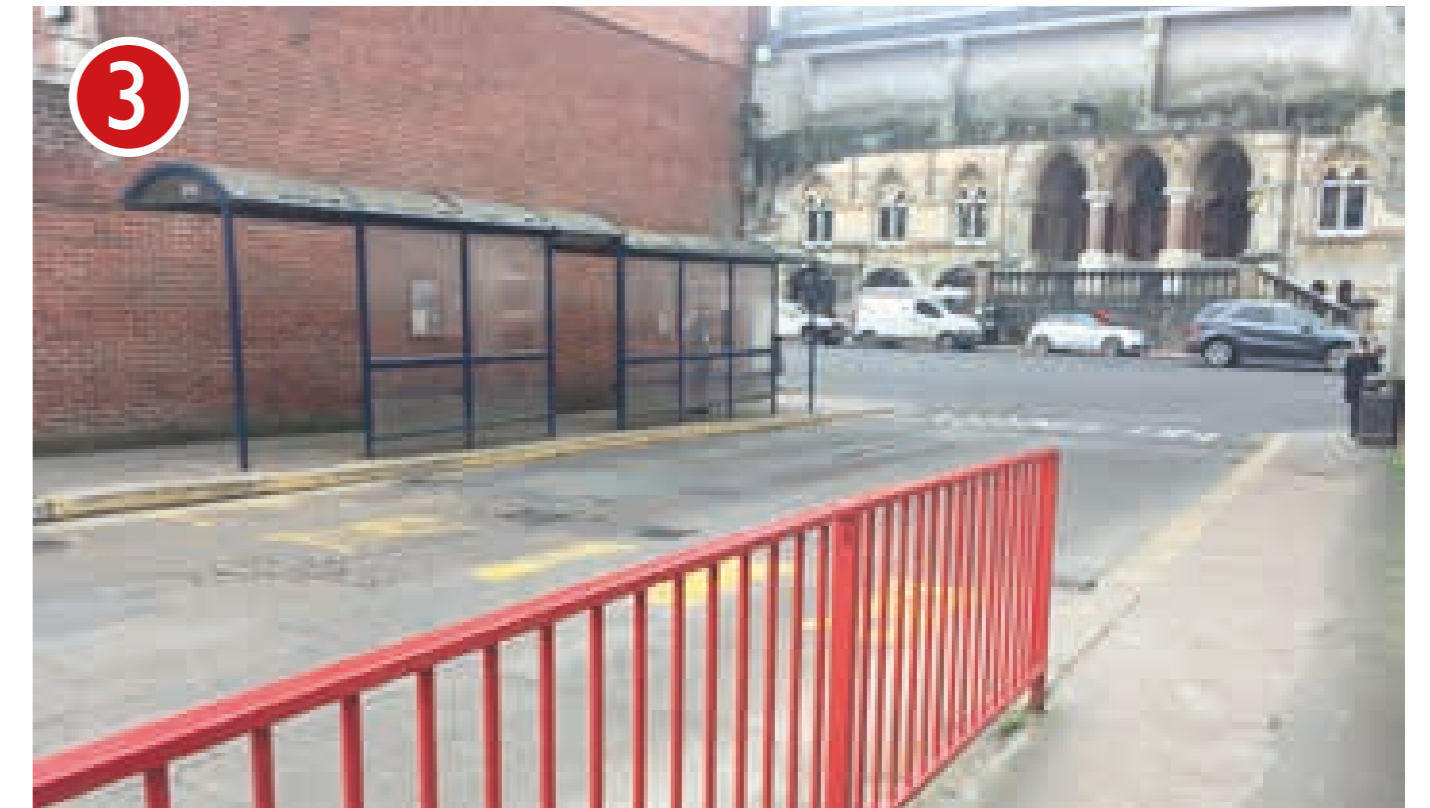
The bus station is not 'pedestrian friendly' with lengths of guardrail giving enclosed and narrow footways with no dropped kerbs or tactile paving.
