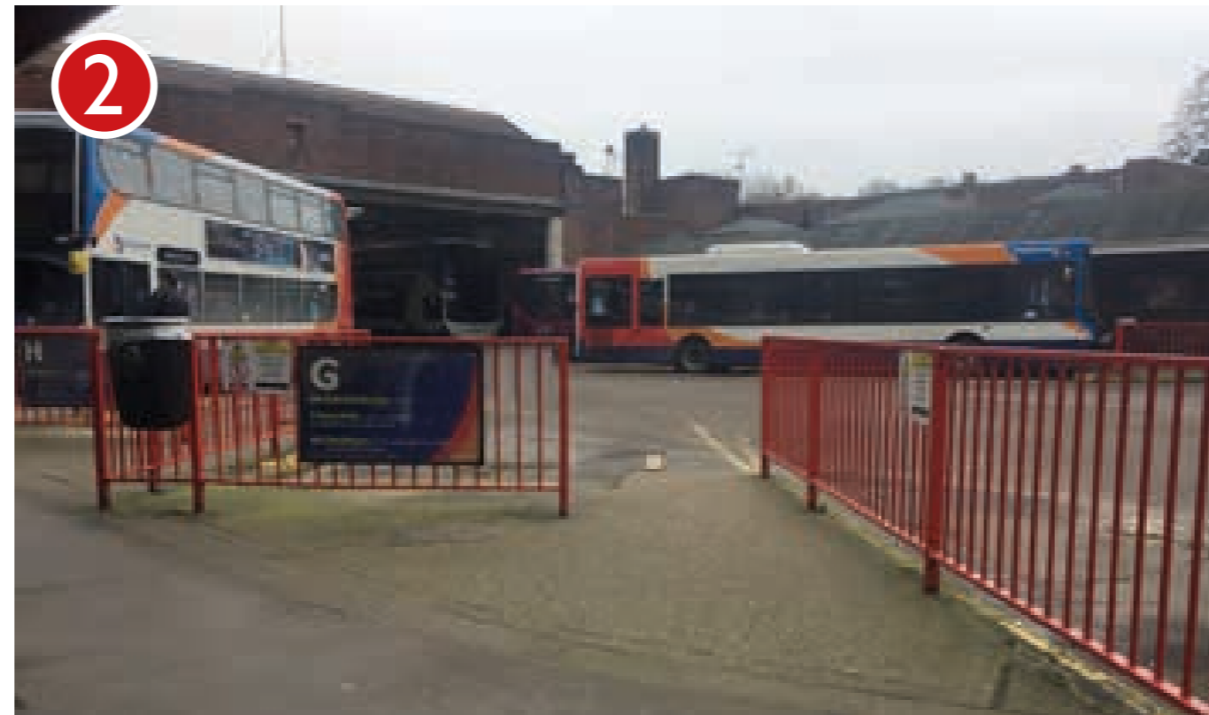
The bus station has a 'tired' and dated appearance.
