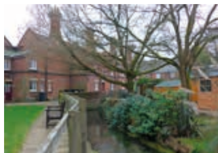
St John's Almshouses boundary wall
