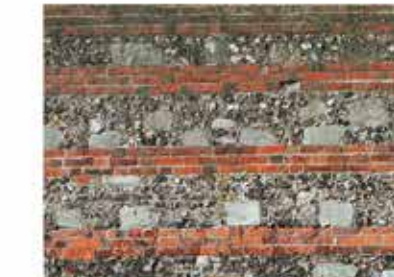
Banded brick with stone flint panels
