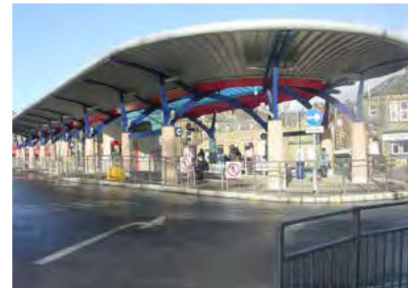
Pudsey's New Bus Station - looking towards Church Lane cc-by-sa/2.0 - © Betty Longbottom - geograph.org.uk/p/2253723
