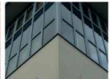
Curtain wall glazing and render
