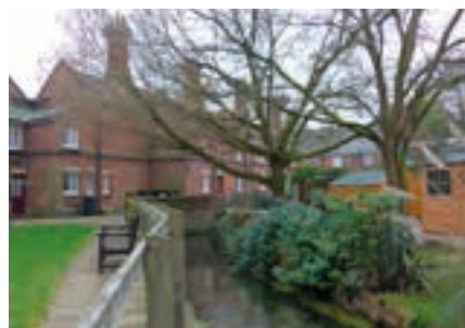
St John's Almshouses boundary wall
