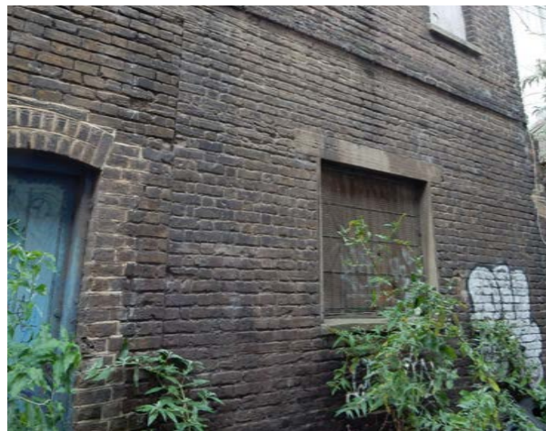
Brickwork, arched openings
