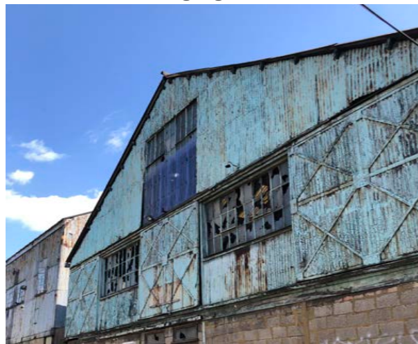
Pitched roof, metal, colour
