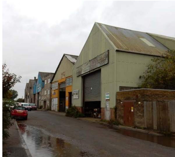
Pitched roof, metal, colour
