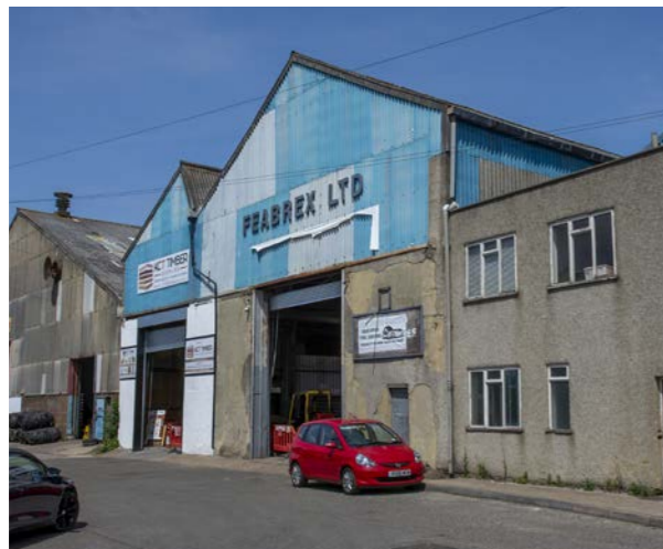
Pitched roof, metal, colour
