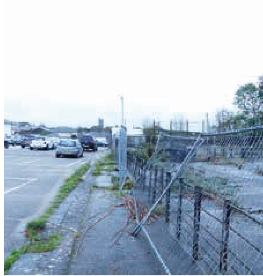
Site photo of surrounding existing structures
