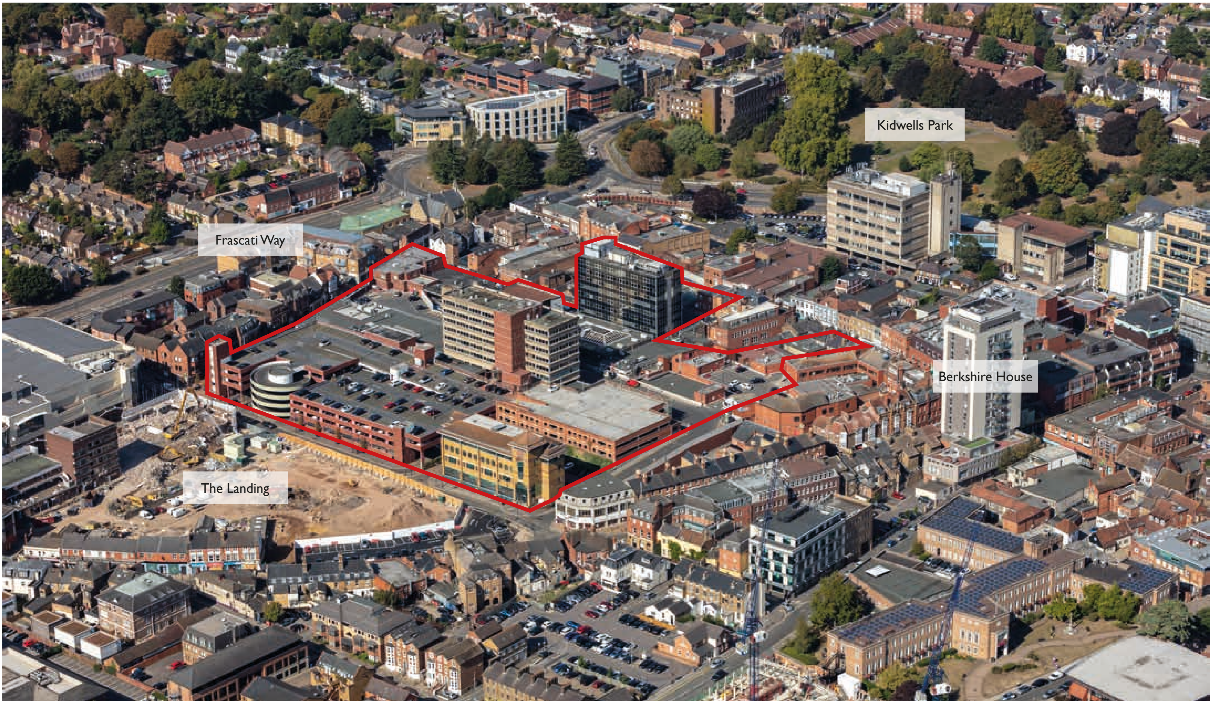
Aerial View from South East
