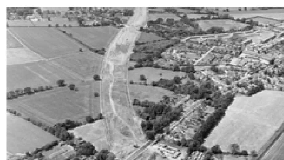
M4 preparation works near Woodley - west of Maidenhead.
