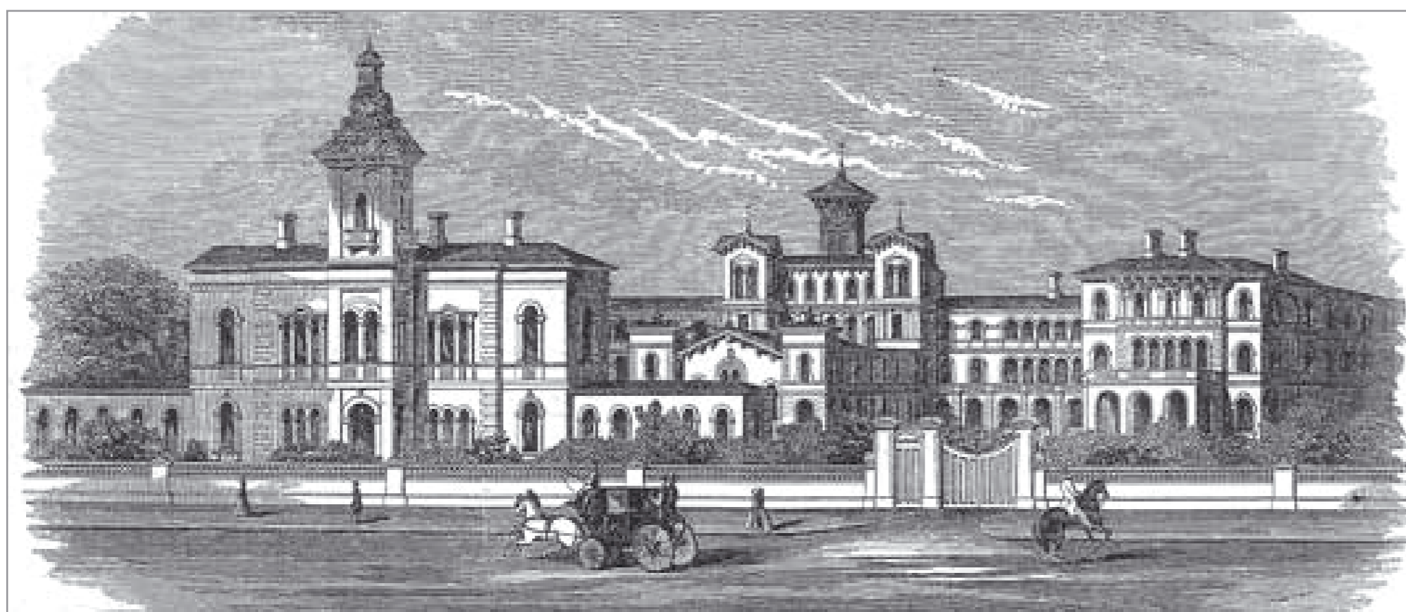
The City of London Union Workhouse perspective drawing illustrated in the Builder 11 August 1849
