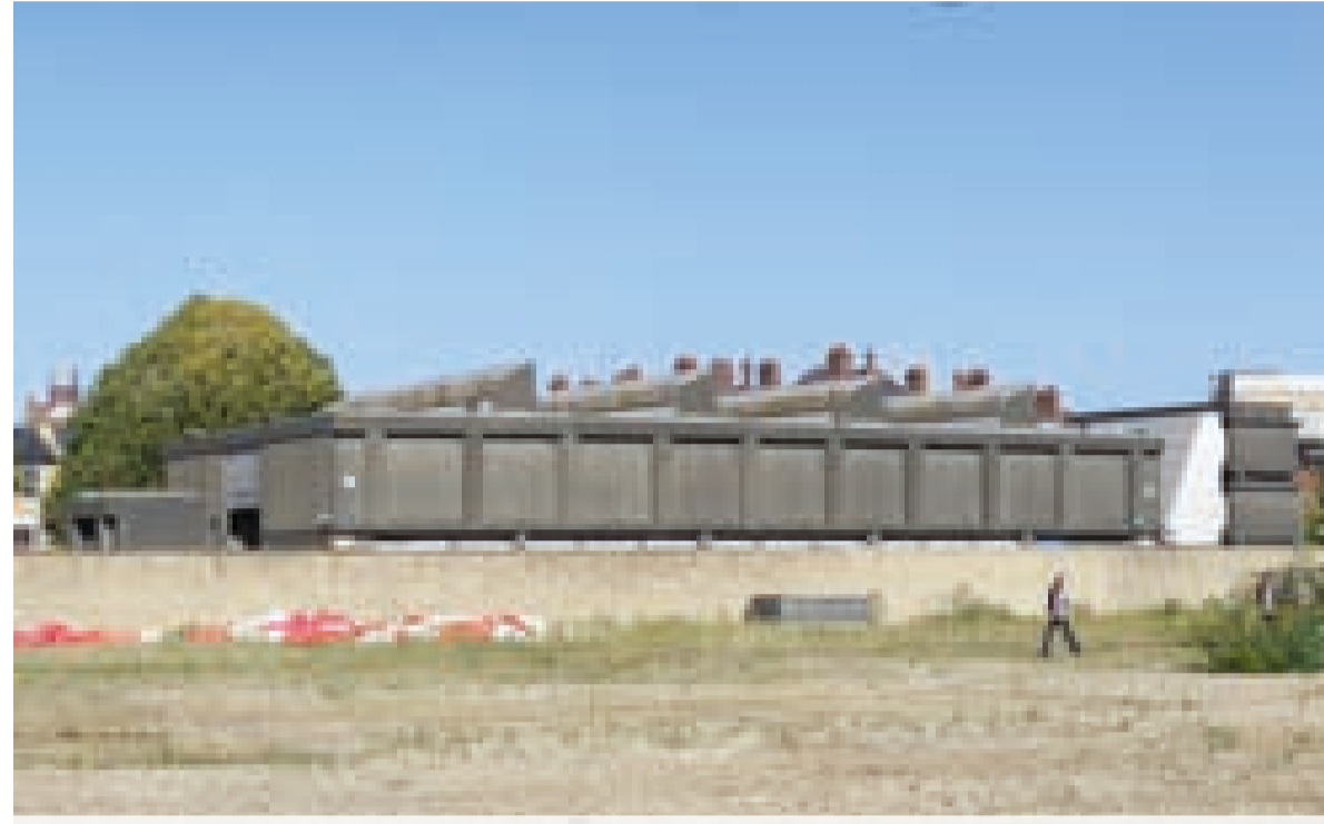
Thames Water pumping station
