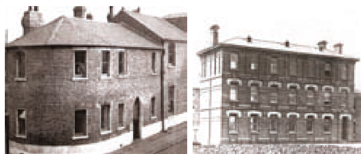
The original cottage dairy - 1876 Fulham Union Infirmary - 1884
