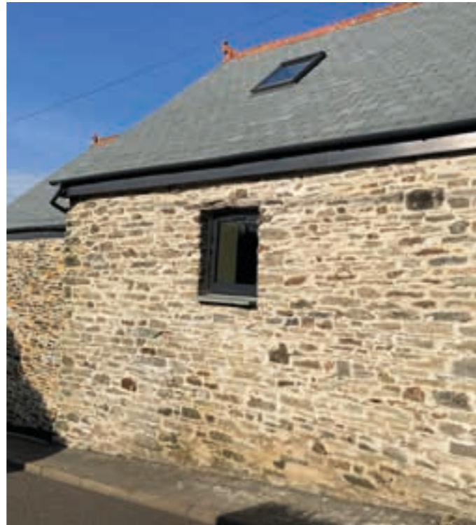
Callywith stone and slate roofs
